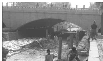
图3 小月河河底防排水施工 Fig.3 Preventing and draining construction of Small Moon River bottom
